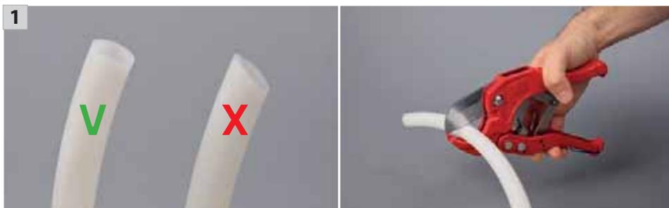
**Pipe cut.** Square-cut the pipe perpendicularly to its axis, using the R990 cutter and taking care not to deform it.
