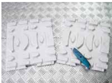
R884 head panels cut to measure
