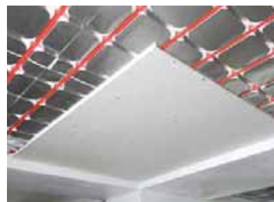
Installation and fitting of plasterboard sheets on the support structure after pressure test performed according to the rules in force
