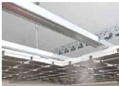
Installation of metal structure with 300 mm pitch
