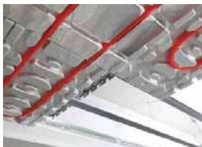
Installation and fitting of R883-1 panels and pipes along the preformed panel and head housings
